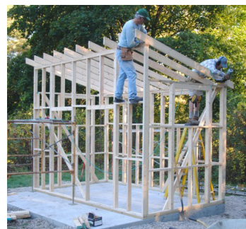
Framing, roofing, siding, windows, done!
